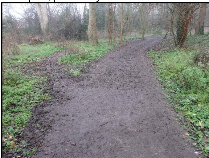
Figure 2 Gravel surface showing beneath mud
